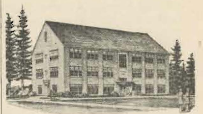
SCIENCE HALL (Under Construction)
