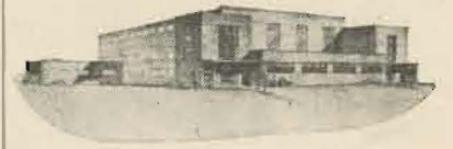
NEW GYM (Under Construction)
