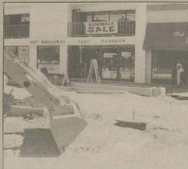
Construction on Broadway Street.
