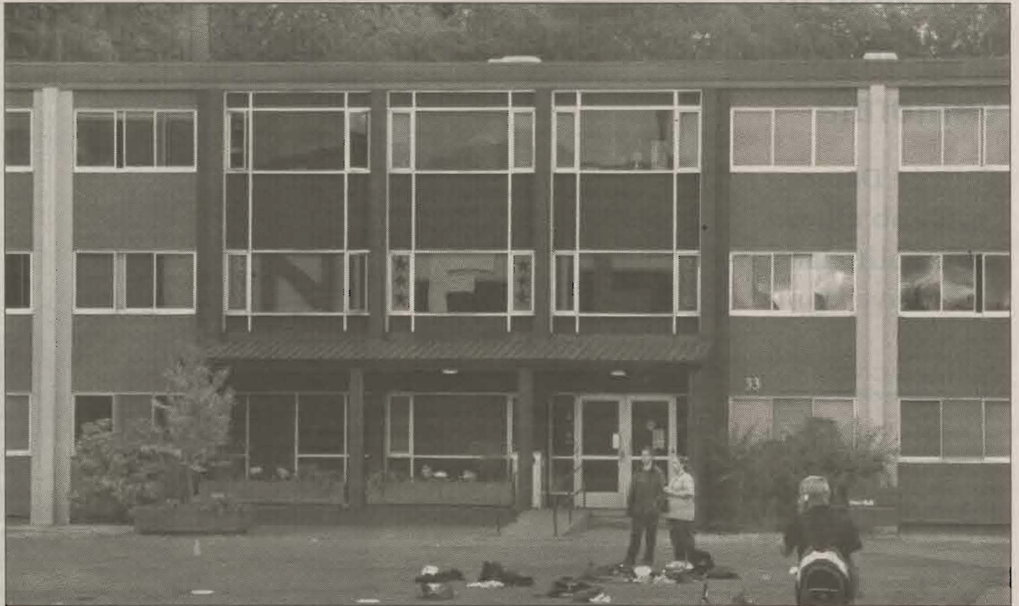
A coat of paint goes a long way: Students socialize in Foss Field in front of the newly renovated Foss Hall. The lower campus residence hall received new burgundy, brown and beige paint colors as well as interior features including new carpeting, hallway lighting and a refurbished front desk area.
