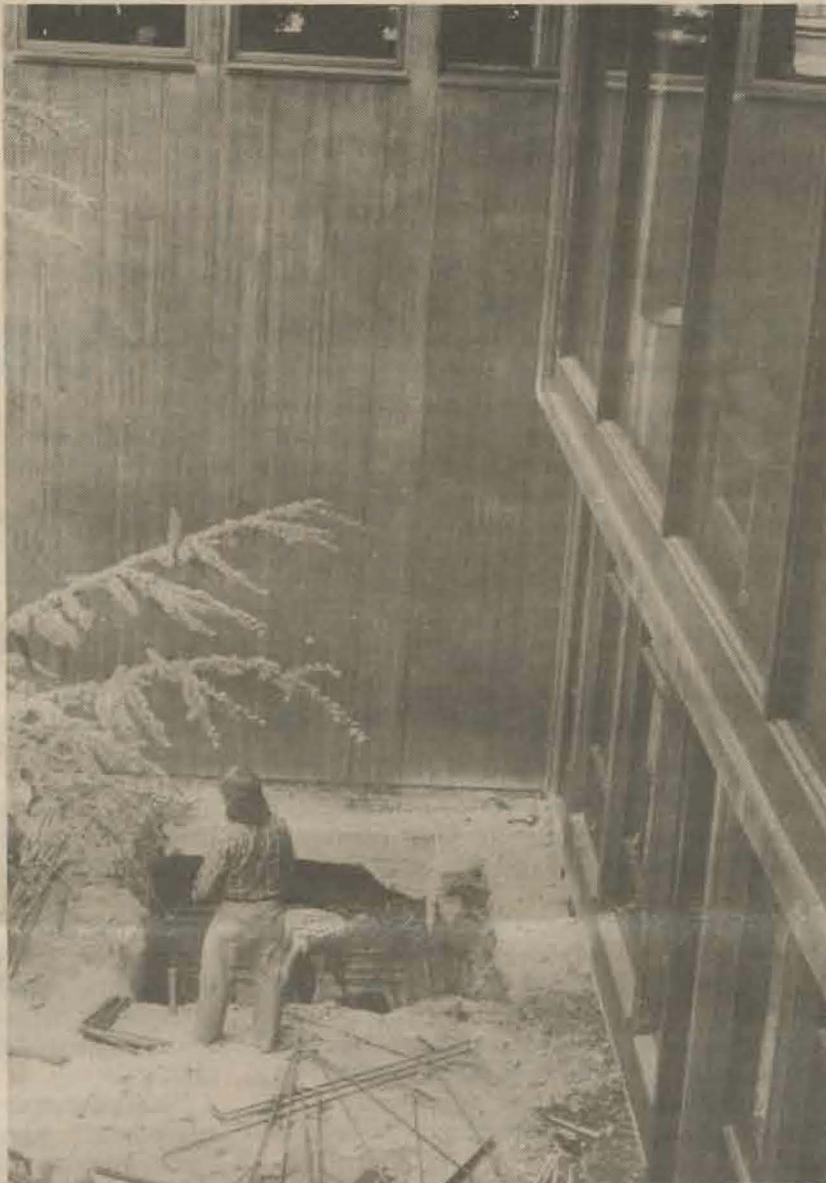
C and T Construction Company is in charge of the job.
