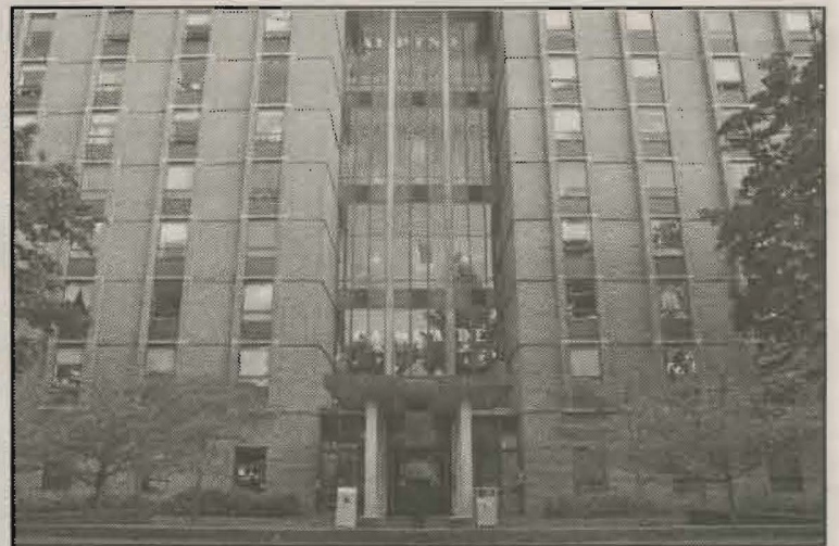
Photo by Chris Hunt Tinglestad Residence Hall before the summer renovations. Contractors plan on the Tinglestad being ready for the fall.
