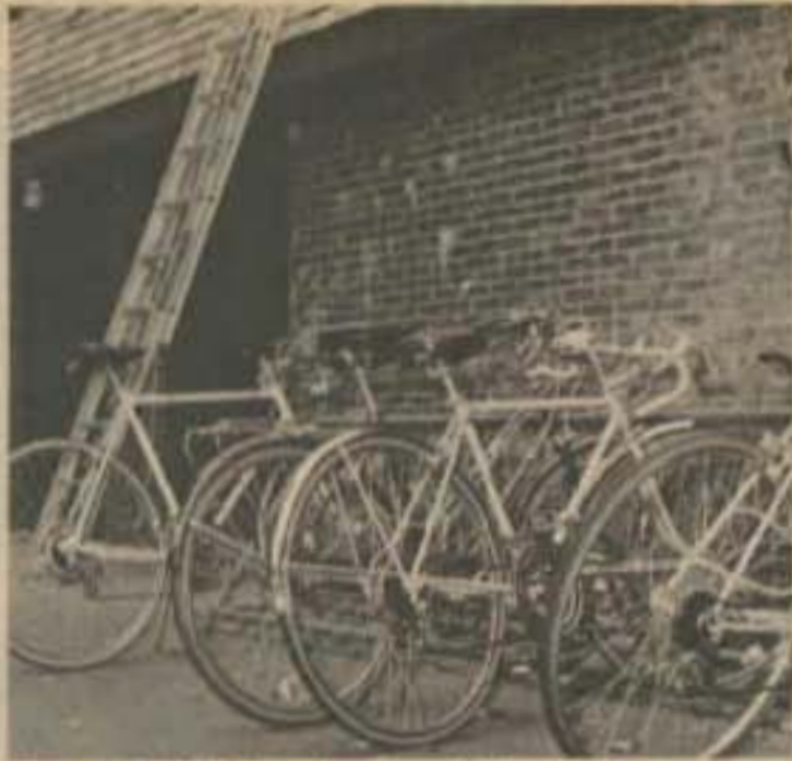
NEW ADDITION: Recently constructed is a bicycle storage room behind Harstad Hall for use by its residents. Maintenance constructed most of the brick structure; it is currently being examined to determine how the most bikes might be stored easily.
