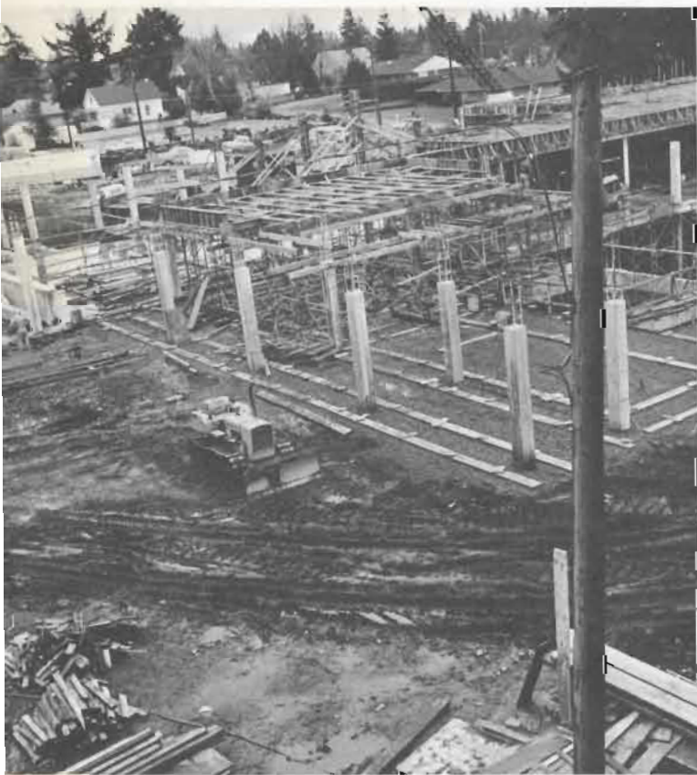
November - Construction continues on the second floor game room area.
