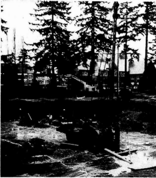
SINKING A CASING —Construction crews are sinking a casing for an emergency drain for the new library. Excavation was completed last week. Earth from the excavation was hauled to other areas of the campus where fill dirt was needed for future parking lots.
