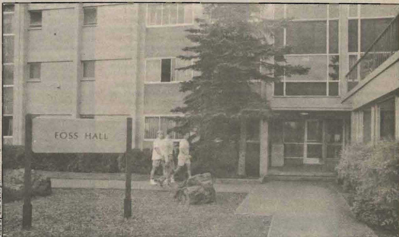
New carpeting, new blinds and a fresh paint job are among the changes that will greet students moving into Foss Hall next fall. The dorm is undergoing major renovation this summer as part of a university plan to upgrade residence halls on a rotational basis.
