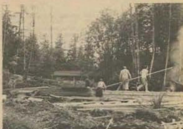
The families involved in "House My People" all work together to build homes for each other.
