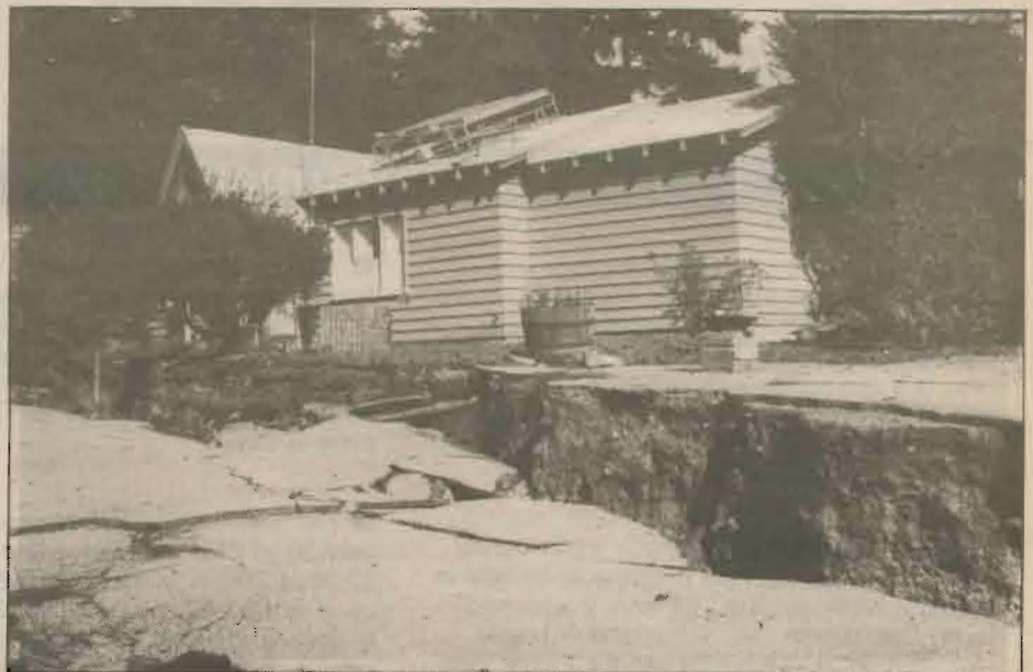
"This crack is not thought to be a fault. Geologists are saying that it is part of an ancient gigantic landslide that the earthquake loosened. This is one of several such cracks in the mountains. The Tranborgers live in the house right behind the crack. The house suffered no major damage and they were back living in the house when this photo was taken, eleven days after the earthquake."
