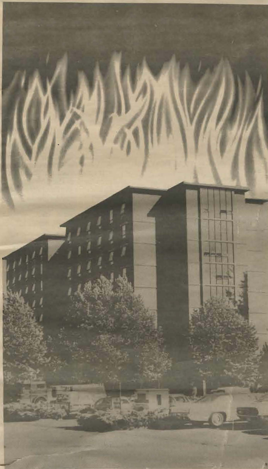
Parkland Fire Chief Les Flue says Tingelstad is a fire hazard
