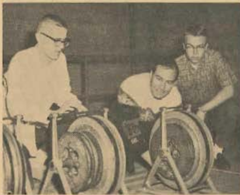
HIGH ABOVE the CMS stage, looking at the flying apparatus which will be used in the production of "Peter Pan," are Ken Johnson; Peter Foy of Hollywood and London, who is here supervising the installation and rigging of the apparatus; and Ron Enger. The Children's Theatre will premier Saturday, March 17, and will be enjoyed by thousands of children from the surrounding area.
