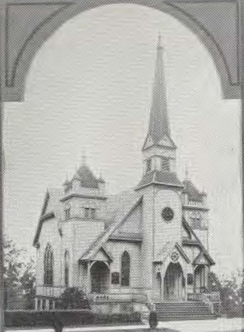
FIRST NORWEGIAN LUTHERAN CHURCH SOUTH TWELTH AND I STREET TACOMA, WASH.
