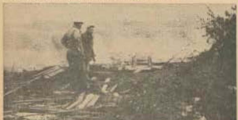
PLU was not alone in its clean-up campaign. The community of Parkland also held a "clean the community" drive. Pictured above is a fire started near Delta Hall to clear away some of the unattractive brush in the area. Parkland firemen also burned down one of the old buildings on Garfield Street in front of Hessel Hall.
