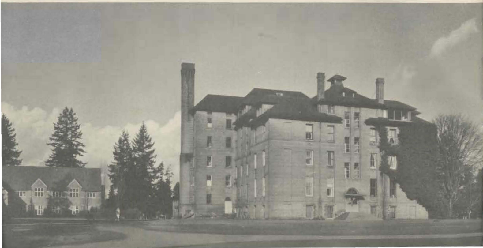
SOUTHWEST SIDE OF OLD MAIN WITH LIBRARY ON THE LEFT
