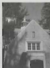
On the cover Xavier Hall, on the PLU campus, is undergoing extensive interior renovation. PHOTOS: CHRIS TUMBUSCH
