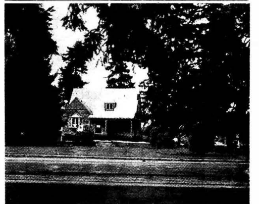
ONE YEAR AGO—This picture, taken last year, shows the site of the new library before construction began. The house shown here, which was later moved, served as the residence of Rev. John Loringgaard, University chaplain.
