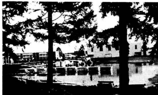
CONSTRUCTION may be said to have dominated these past four years. This year's senior class witnessed the construction of Foss, Stuen, Tingelstad and Ordal Halls as well as a new pool and library.
