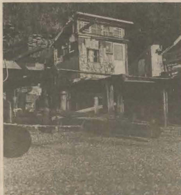
Salmon Beach homes built on piers.
