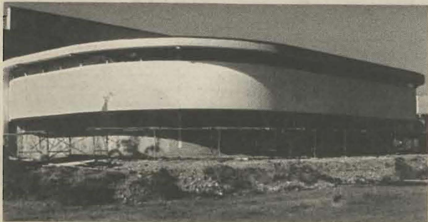
Names Fitness Center under construction
