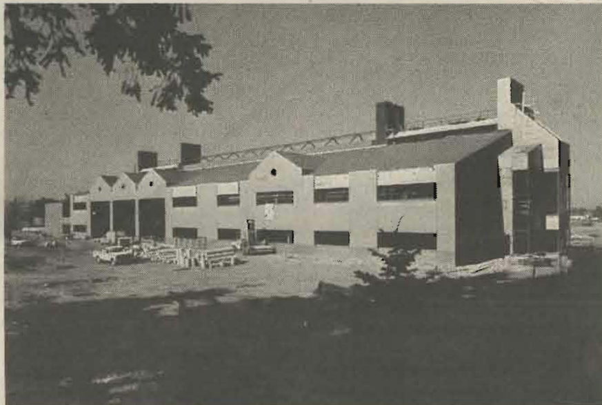
Rieke Science Center in progress
