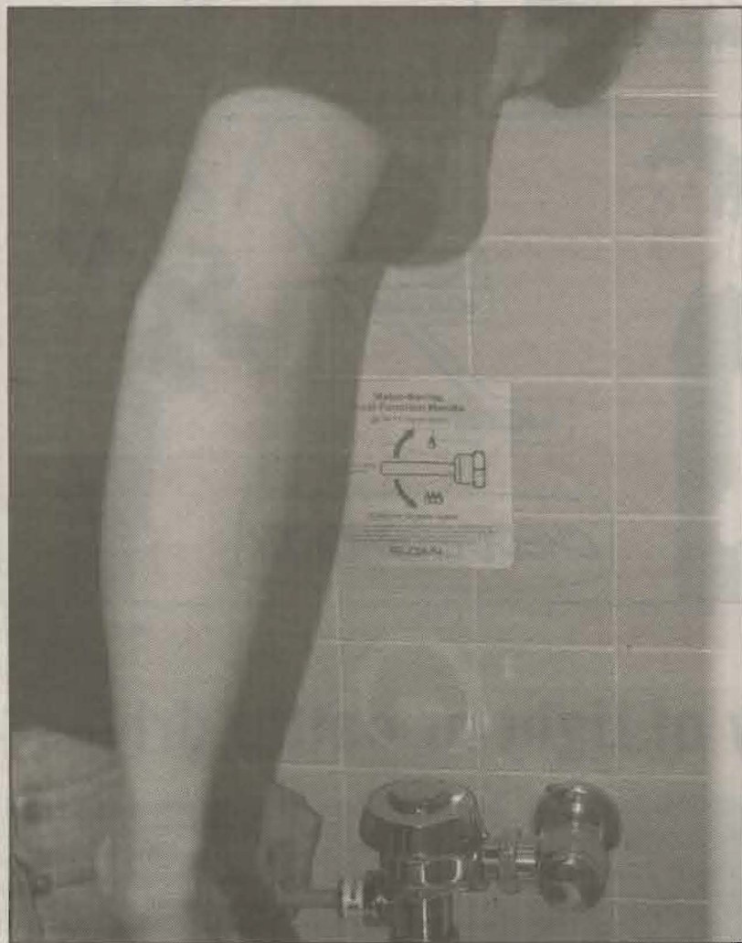
Water conserving toilets are one of the new additions to Pflueger Hall this fall. If the flushing handle is pulled upward the toilet will use less water and pressure than if pulled downward.
