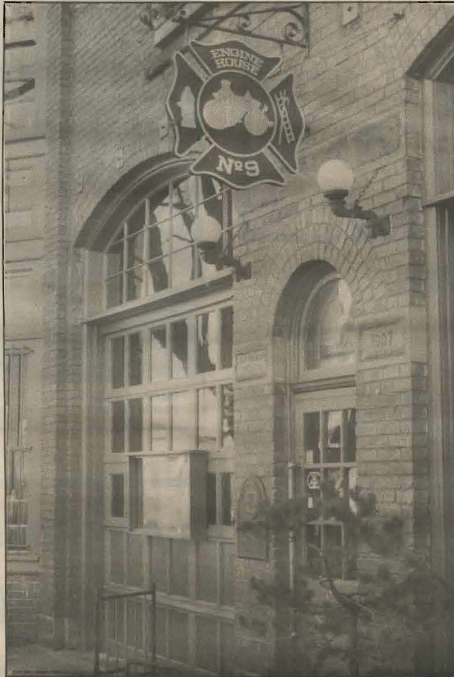
Engine House at 611 N. Pine Street in Tacoma.
