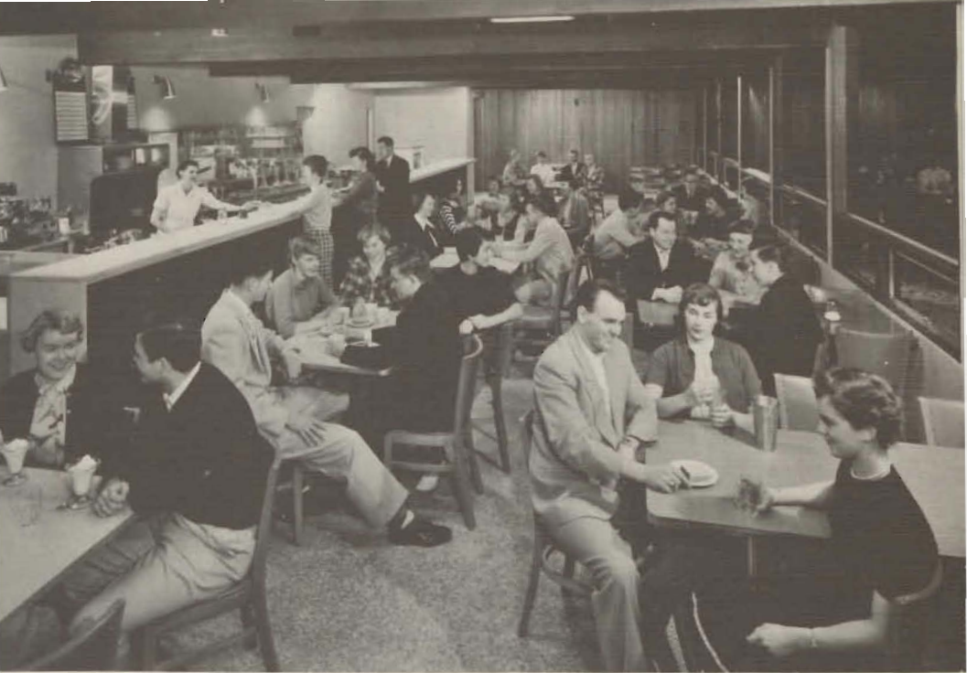
COFFEE SHOP — COLLEGE UNION BUILDING
