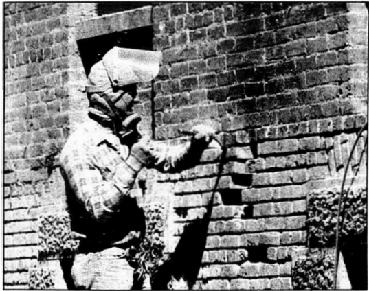
Summer renovation included clearing ivy from the walls of Harstad Hall.
