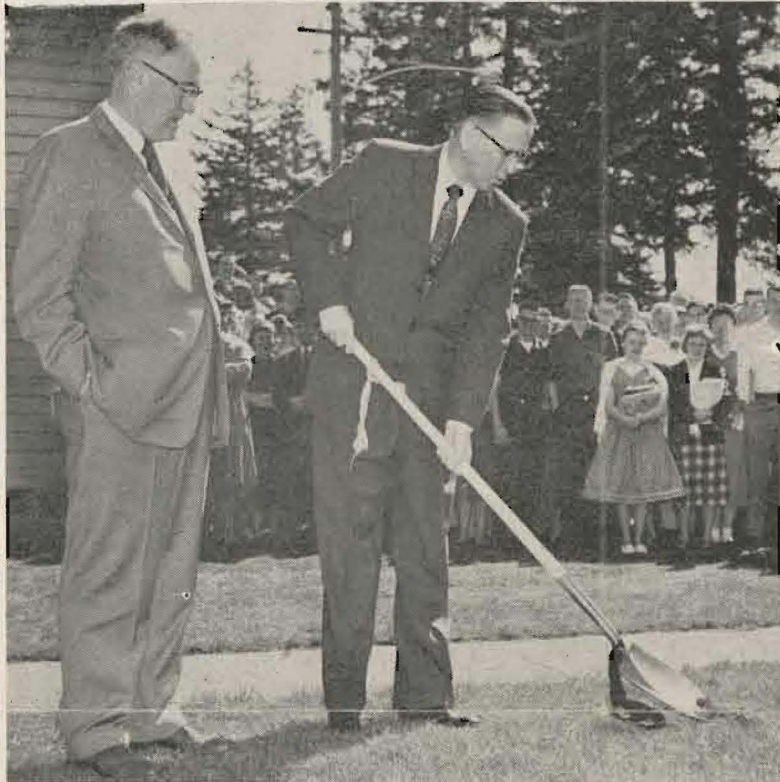
GROUND BREAKING—Dean Philip E. Hauge, member of the faculty since 1920, breaks ground for the new administration building at ceremonies held recently. Looking on, left, is President S. C. Eastvold.
