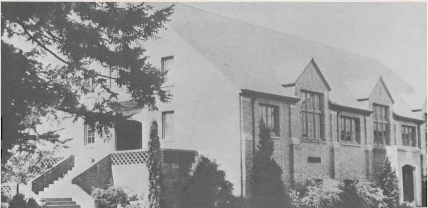
This is the old classroom building, which was later converted to a student union. It stood on the present site of the new student union building.
