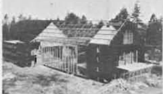
The construction of Eastvold Chapel.
