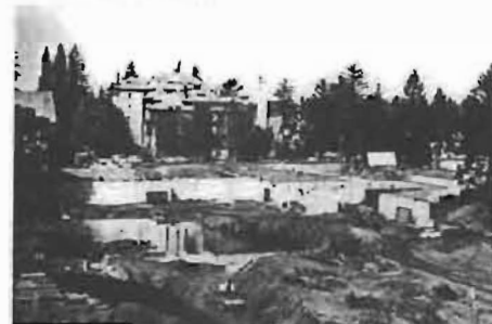
University Center rises on site south of Harstad Hall.
