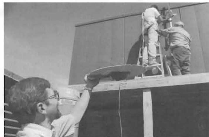
GOING GLOBAL: Peter Winderling, scientific instrument engineer in PLU's Division of Natural Sciences, hands the dish for PLU's new GPS (Global Positioning System) to workers perched atop the Rieke Science Center (summer 1997). The 18-inch pancake-shaped dish boasts a 12-channel receiver connected to a computer inside the science center. Paid for by a grant from the Kresge Foundation, GPS enables students and faculty to find very precise locations in terms of latitude and longitude, which is helpful in research and map making.
